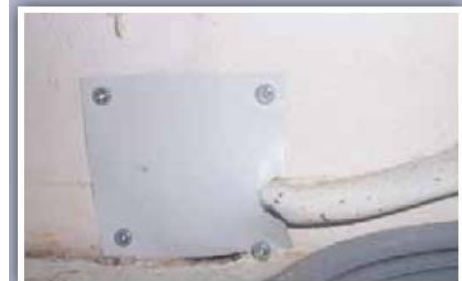
Power supply hole sealed with metal flashing.*
