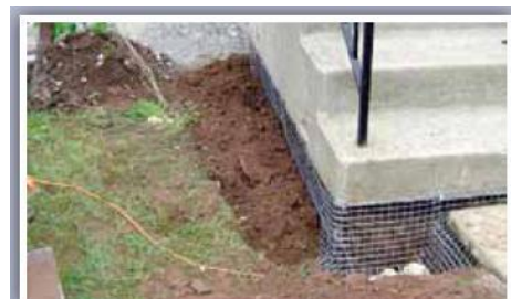
L-Shaped screen application around foundation.***
